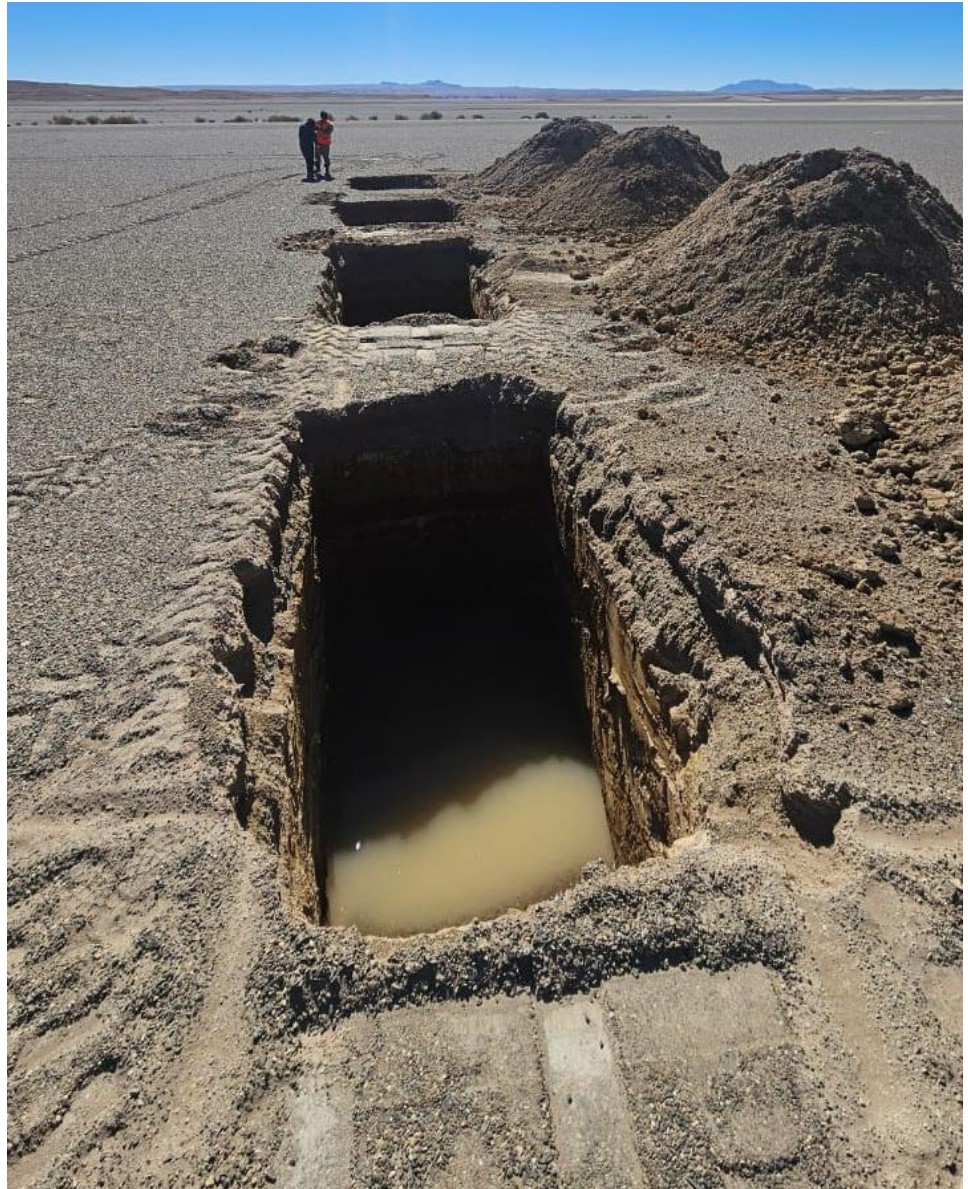
Figure 1. Well JAM 25-05 salt water drill sump holes.
