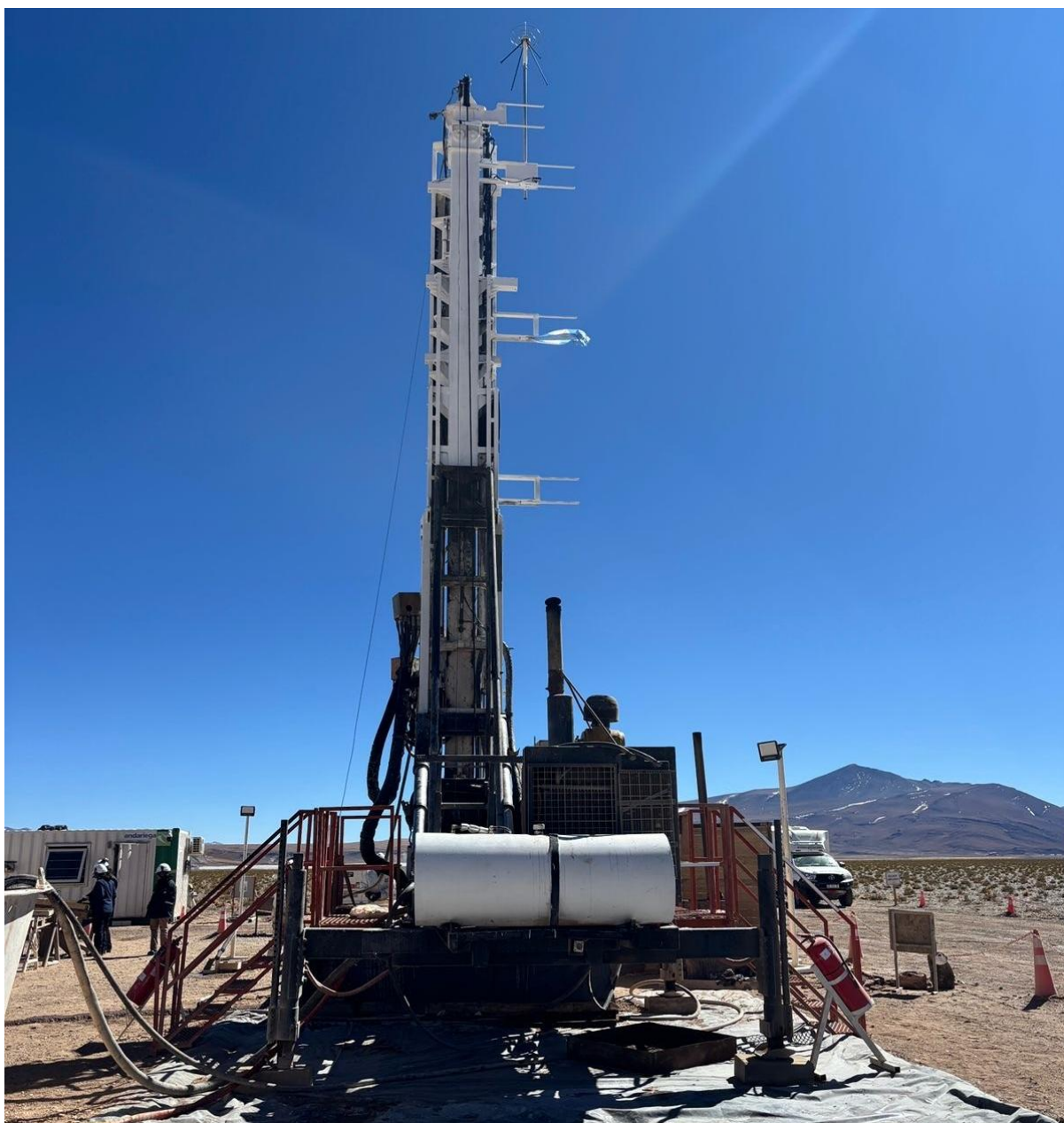
Figure 5. Drill rig that we will drill Formentera JAM 25-05
