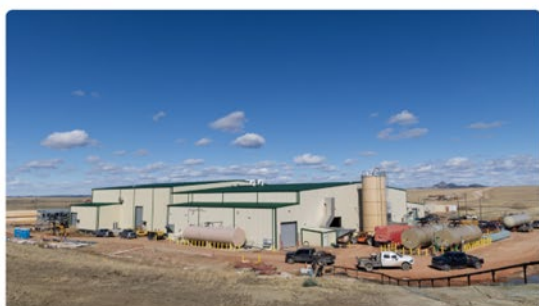
Central Processing Plant (Phase I & II)
