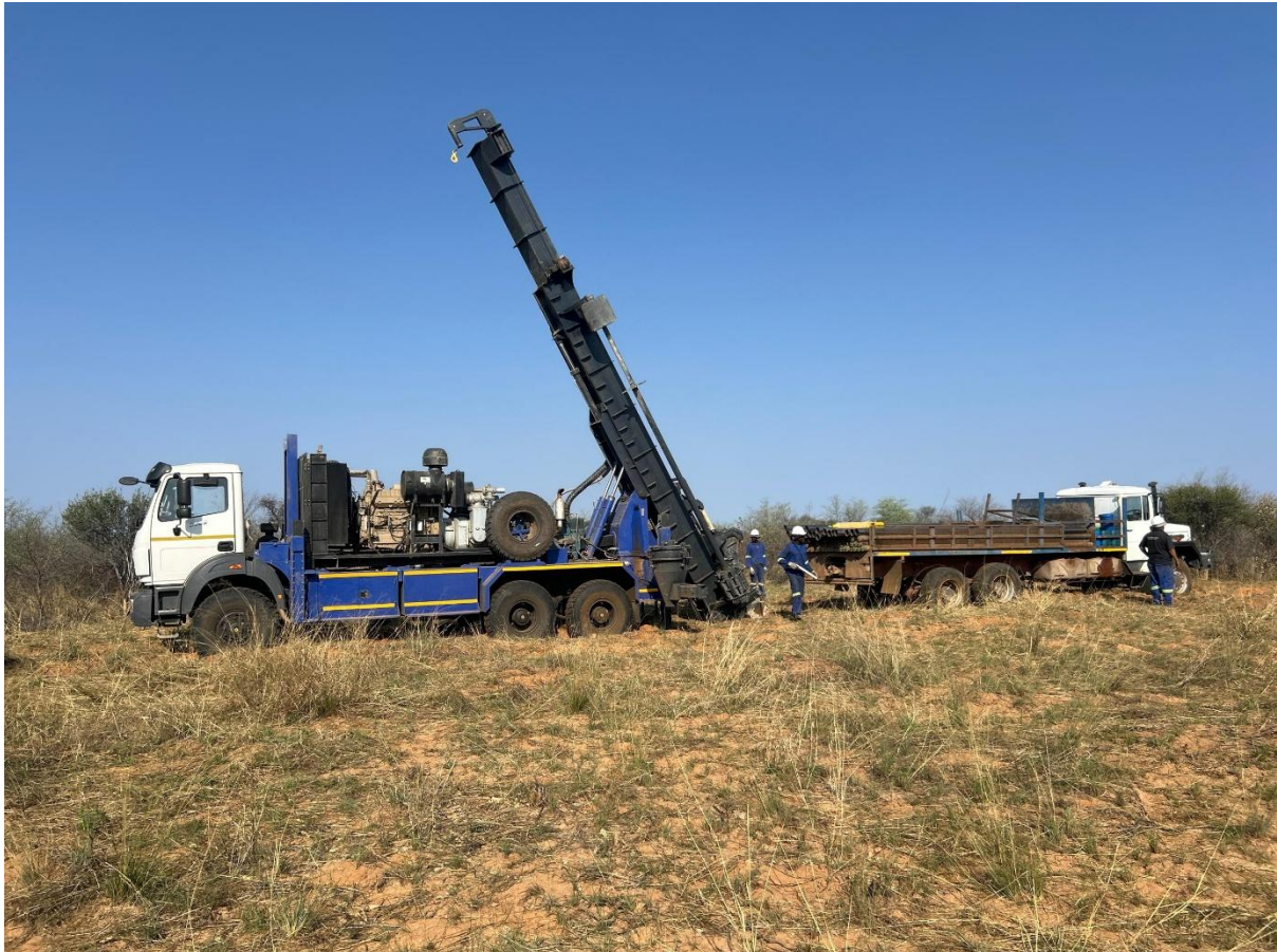
Figure 5: RC drilling commences at the Powerline Project.
