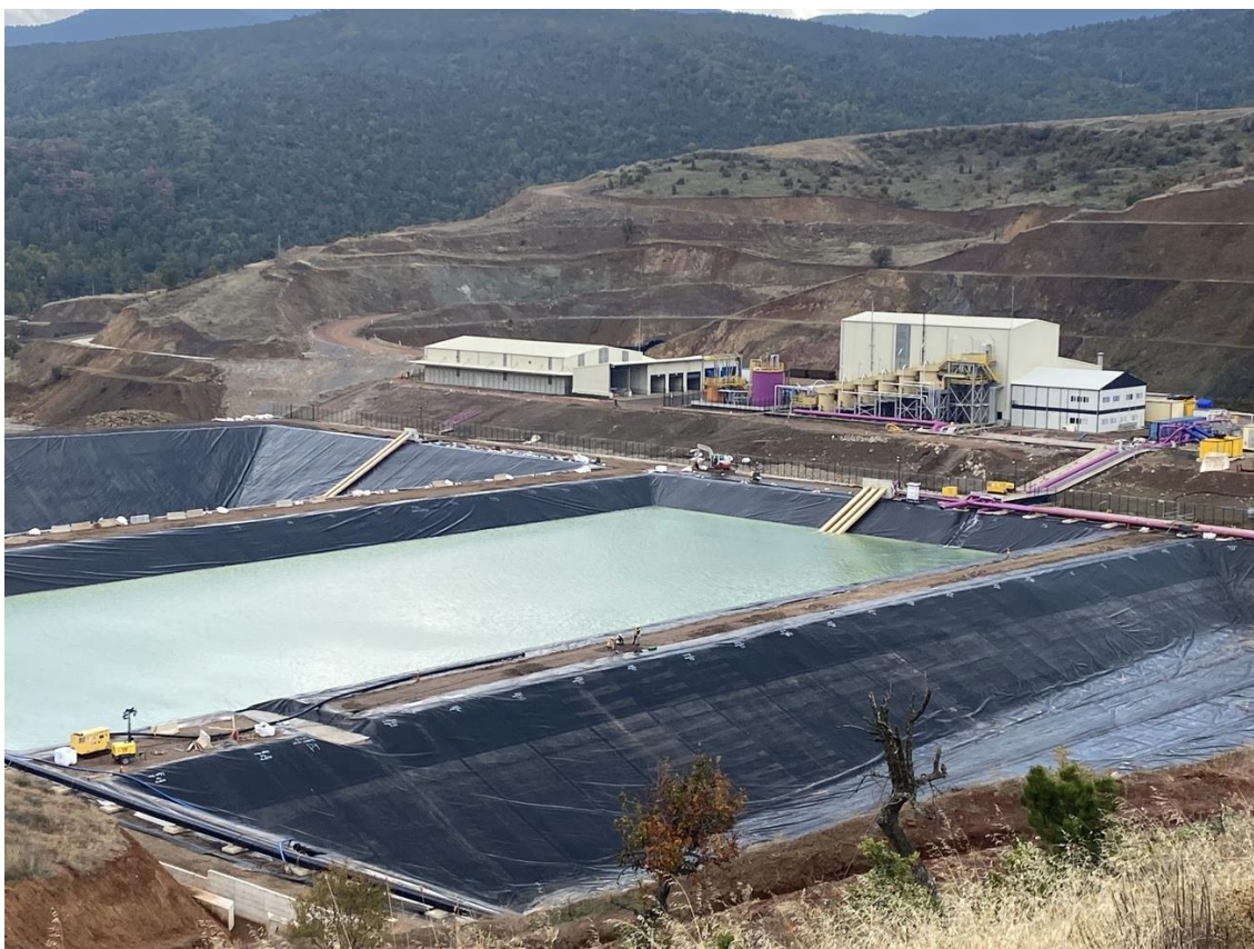
Figure 3: Tavsan heap-leach processing plant and processing water ponds. Photograph taken in October 2025.
