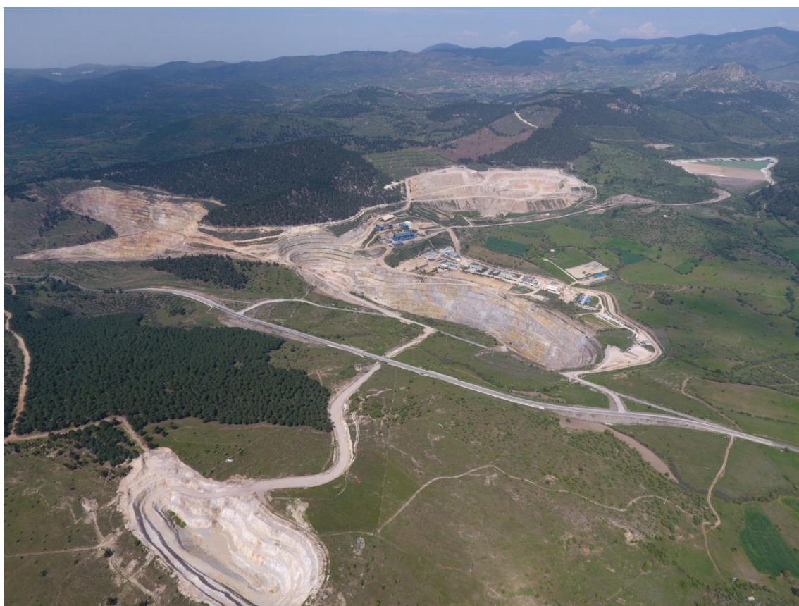
Figure 2: Kiziltepe gold-silver mine showing the open-pits at Arzu South, Arzu North, Banu and Derya, the CIL processing plant (in blue), waste rock dump and tailings dam (in the background). Photograph taken in September 2025.
