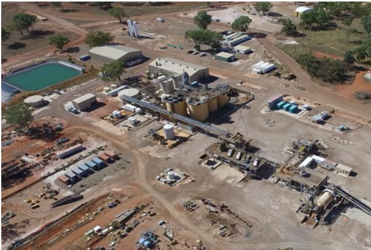
Figure 3: The existing Wonawinta Processing Plant.
