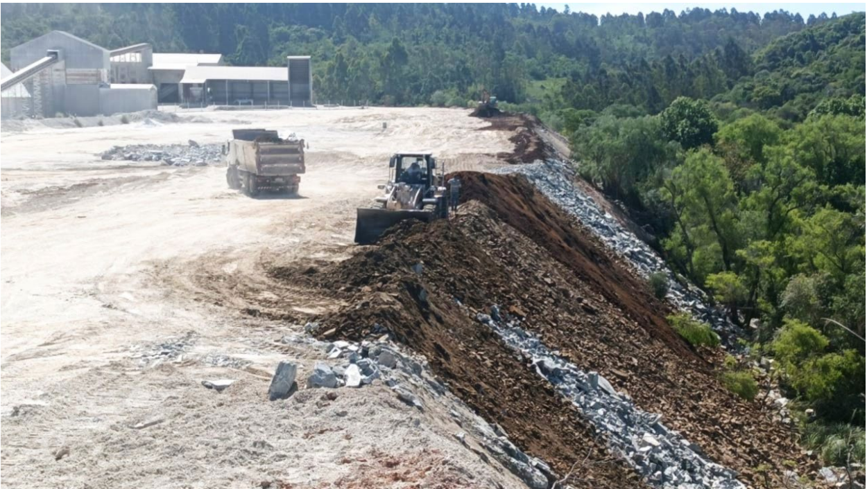
Photograph 4: Civil construction of access road and infrastructure site. Aguiá PAMPAFOS plant in the background.
