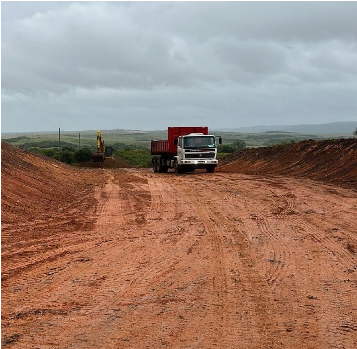
Photograph 5: Construction of the mine access road at Tres Estradas mine site.
