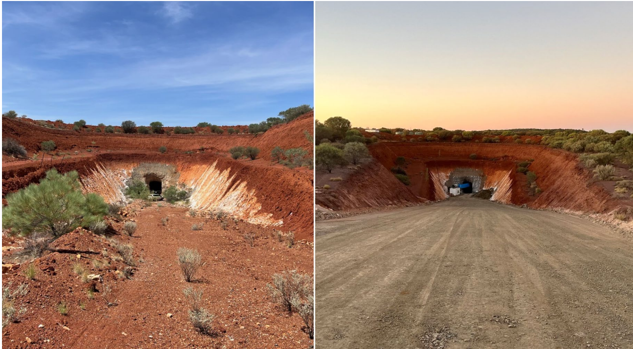
Figure 8: Refurbishment of K2 boxcut and portal
