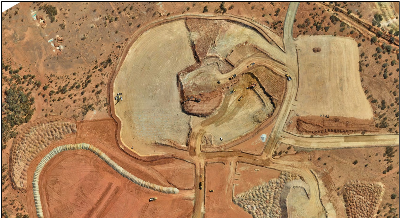
Figure 7: Trident open pit progress during September
