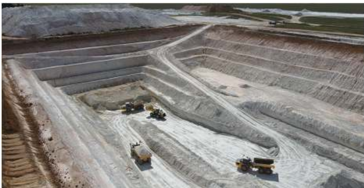
Figure 2: Pit expansion towards into the eastern lode of the Wickepin deposit
