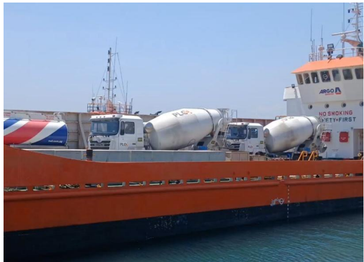
Deployment of Equipment at Wharf
