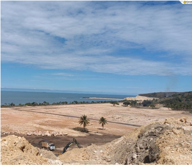
Site Grading and Grubbing for Civil Works Preparation
