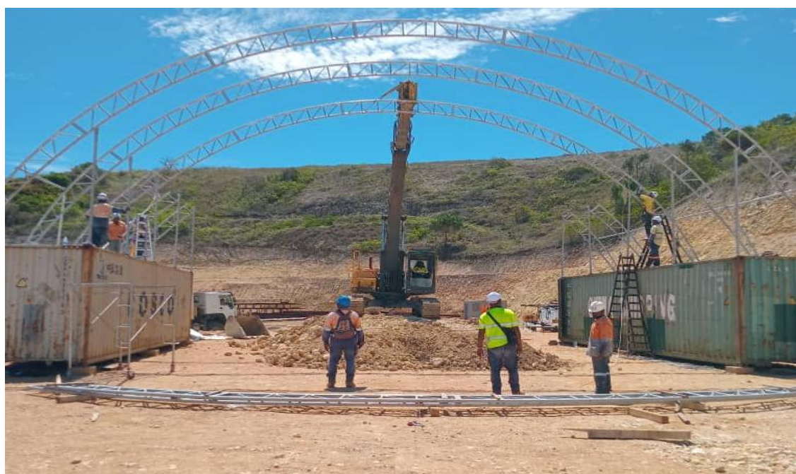
Construction of Workshop Area
