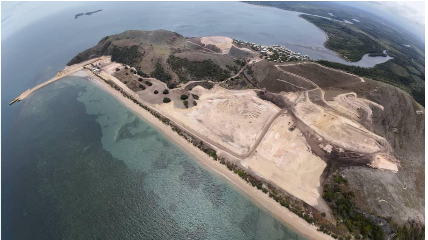
Photo – Aerial view showcasing ongoing construction activities and site preparation works.
