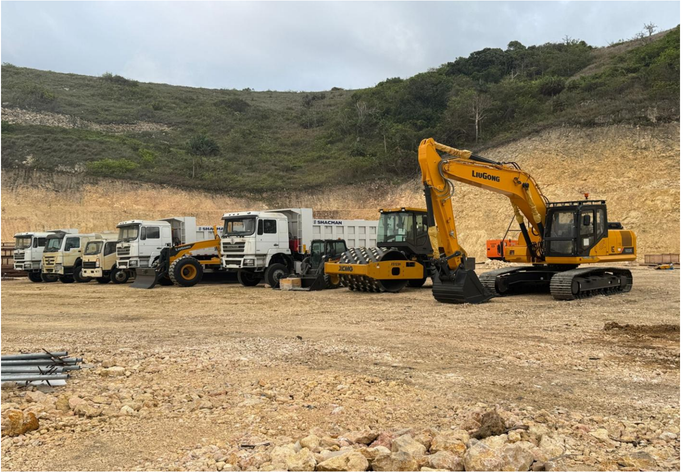
Photo – Pacific Lime and Cement’s construction fleet mobilised on site as works progress.
