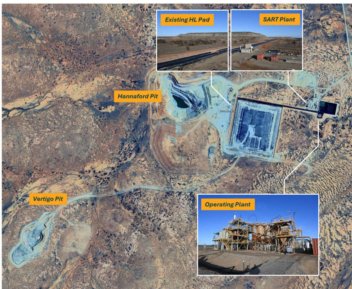
Figure 4: Aerial view of White Dam gold operations site with photos of existing operating infrastructure and heap leach pad.
