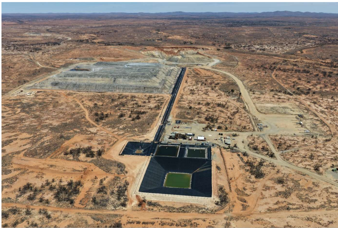
Figure 1; Drone captured image of the current White Dam heap leach facility
