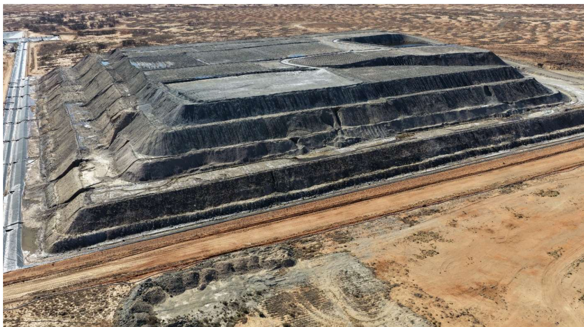
Figure 2; Photo of existing pad looking east, approximately 7.5Mt or ore loaded to date
