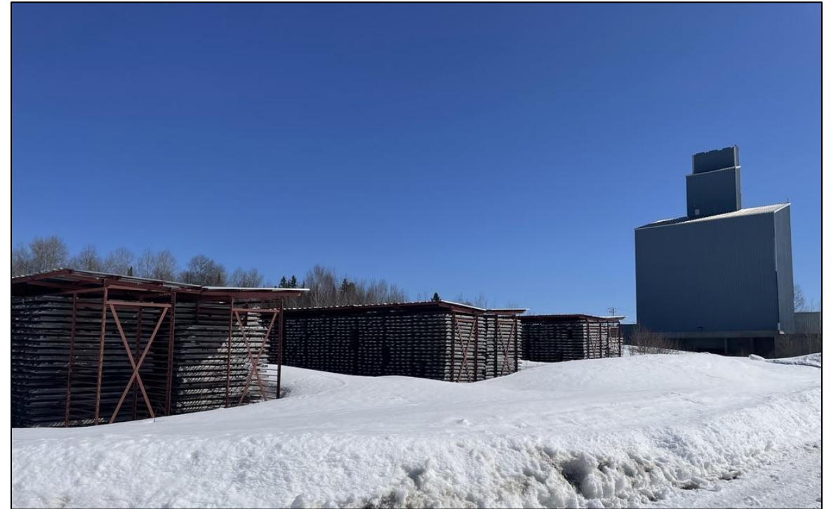
Rouyn Gold Project, Québec. Augmitto site head-frame building & core racks
