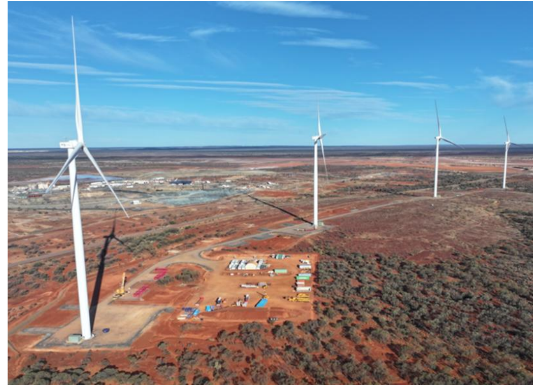
24 MW Windfarm – turbine installation
