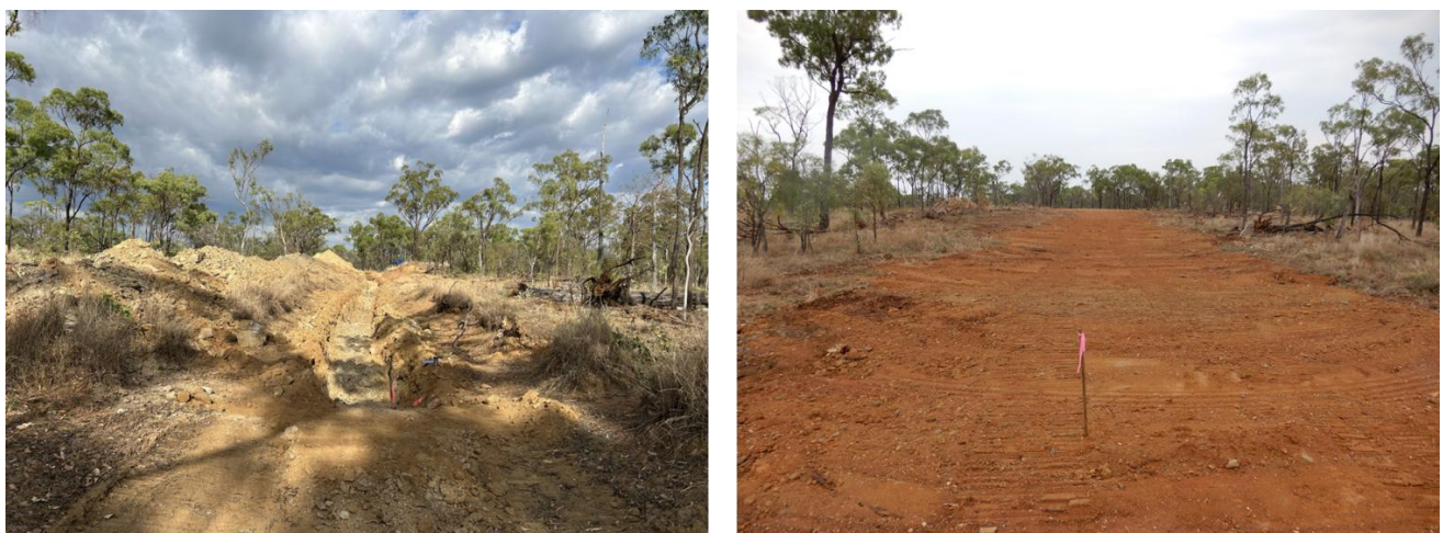
Figure 4 – Greenvale trench 25GRVT04 and the site of an old, exposed trench (ca. 1970s) (left hand image) now fully rehabilitated (right hand image)
