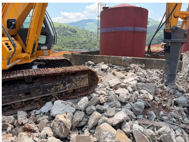
Figure 7: Removing old engineering structures
