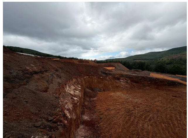
Figure 4: Bulk excavation - gold room platform
