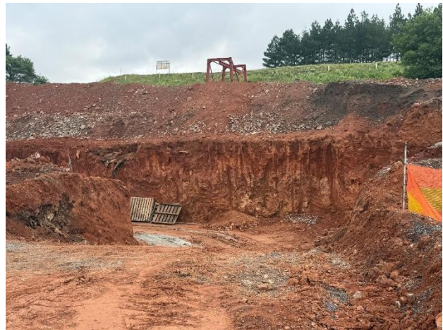
Figure 2: Bulk excavation - concrete retaining walls
