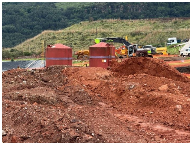
Figure 3: Bulk excavation - platform 4
