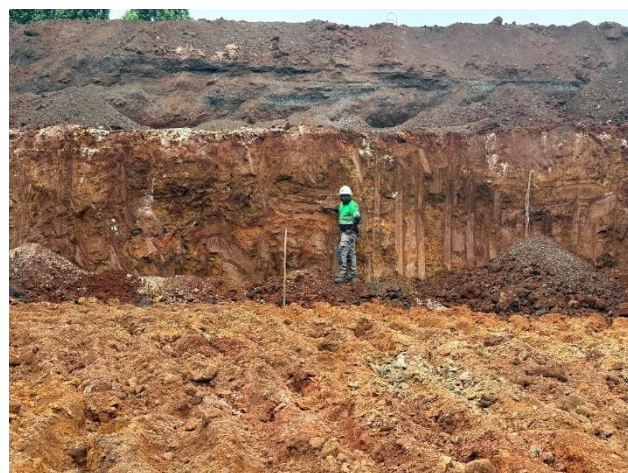
Figure 5: Bulk excavation - gold room platform
