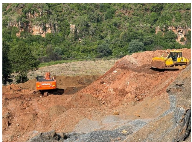
Figure 6: Bulk excavation - platform 3 area
