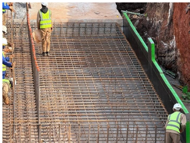
Figure 10: Retaining wall foundation steelworks
