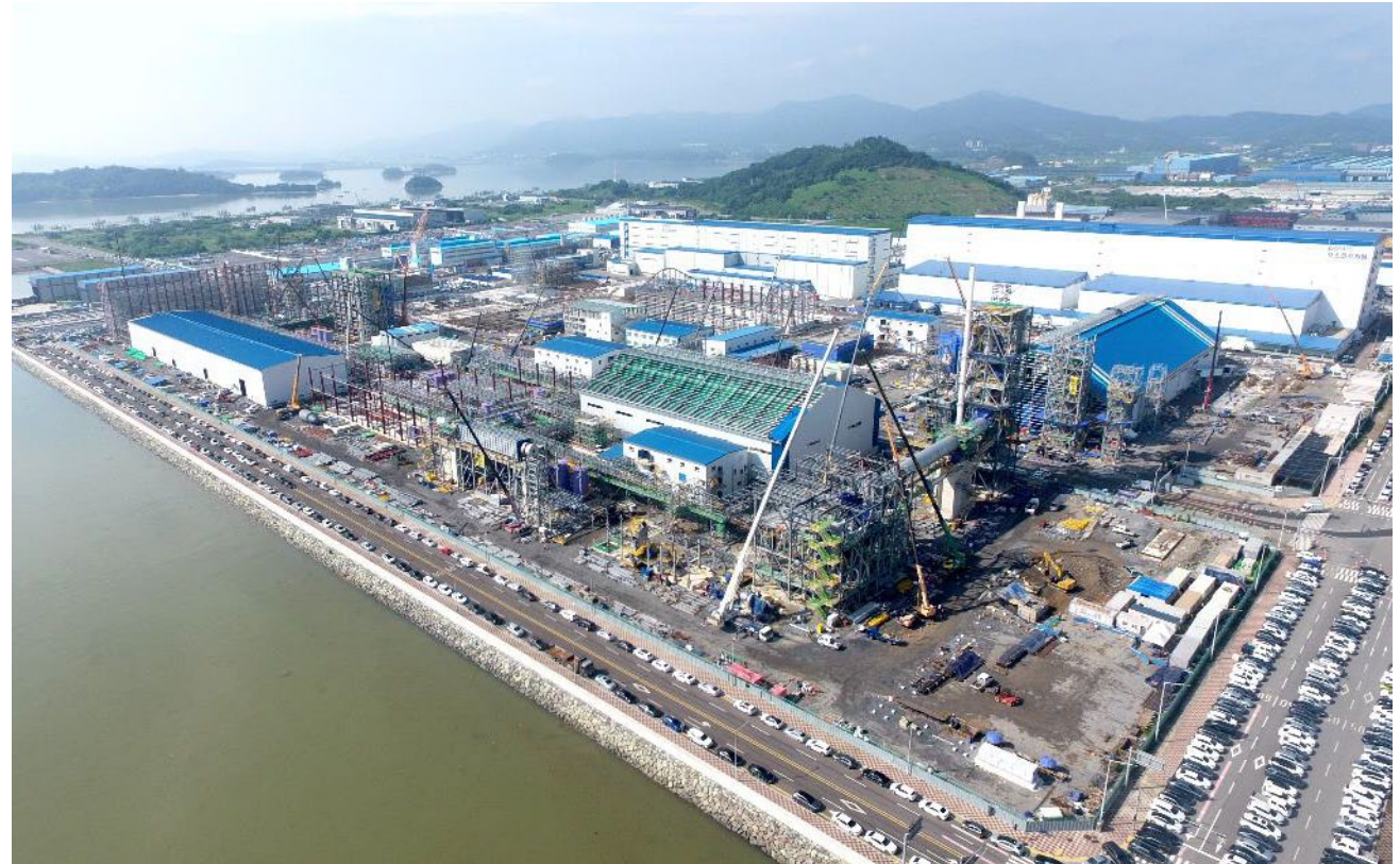
Construction site at the POSCO Pilbara Lithium Solutions LHM facility as at 20 July 2023
