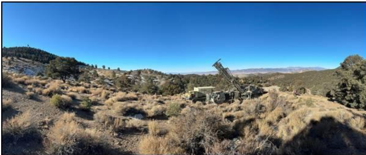
IMAGE: Drilling at White Caps Project, February 2025
