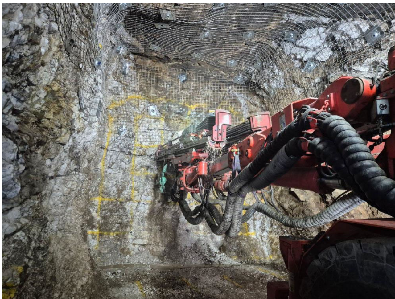
Figure 1: Jumbo development has commenced ahead of schedule, shown on the 1146 East Ore drive.
