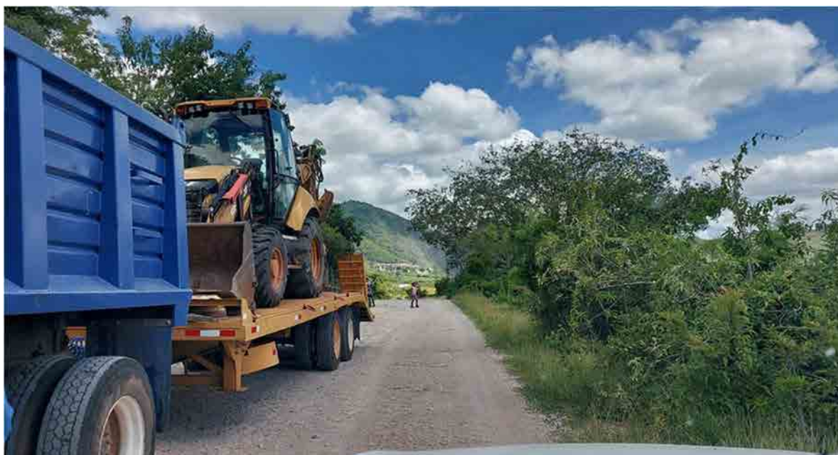
Road infrastructure machinery mobilized. Work commenced.
