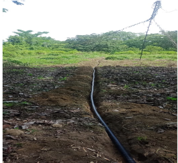
Construction of new 5.5km water pipeline to the Santa Barbara processing plant
