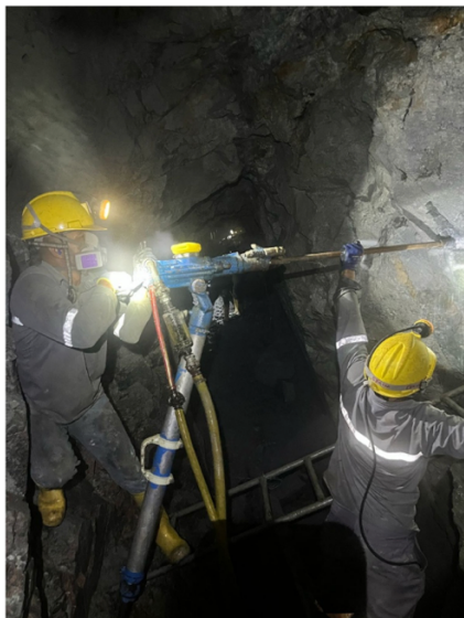
Underground development blasting operations, Santa Barbara gold project
