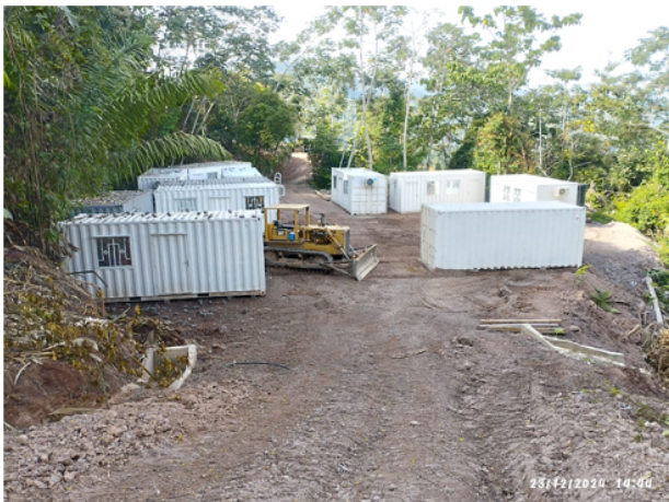
Modern containerised camp being constructed, Santa Barbara
