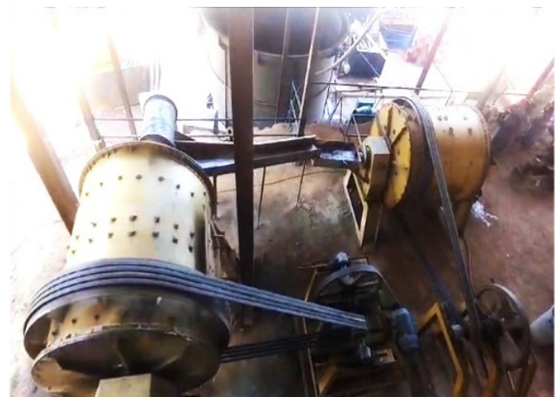
Milling circuit, Santa Barbara processing plant
