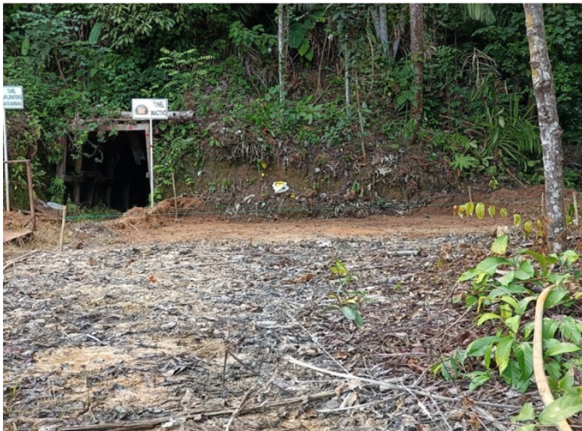
Santa Barbara adit pre-redevelopment, September 2024
