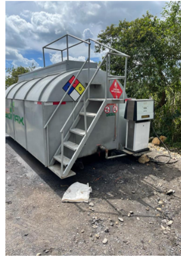
A 5,000-gallon diesel tank is currently being installed for on-site power generation and for diesel vehicles and equipment
