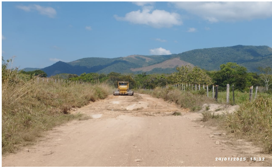
Upgrading of roads between local communities
