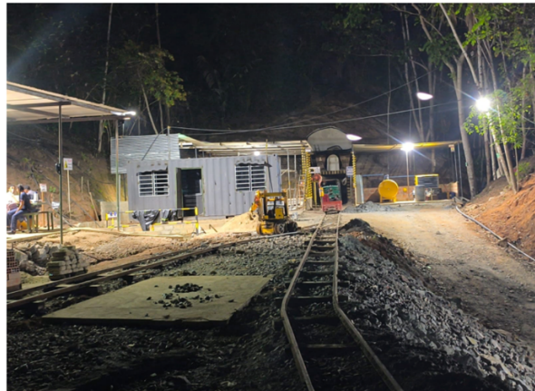
Santa Barbara adit mid-April 2025
