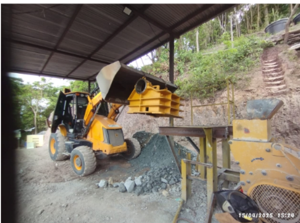
Installation of the new secondary jaw crusher and tertiary crusher, Santa Barbara processing plant April 2025
