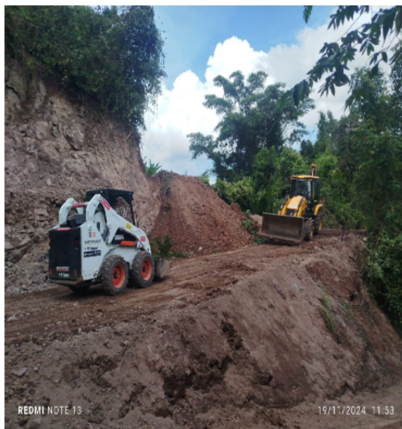
A backhoe/FEL, bobcat and 20 tonne dump truck were purchased early in the construction phase to support civil works on site and to provide capacity to load mineralised material at the adit for transport to the processing plant.
