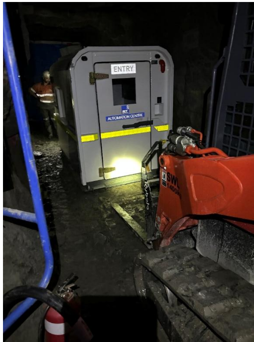
Figure 3 Tele- hut installed underground
