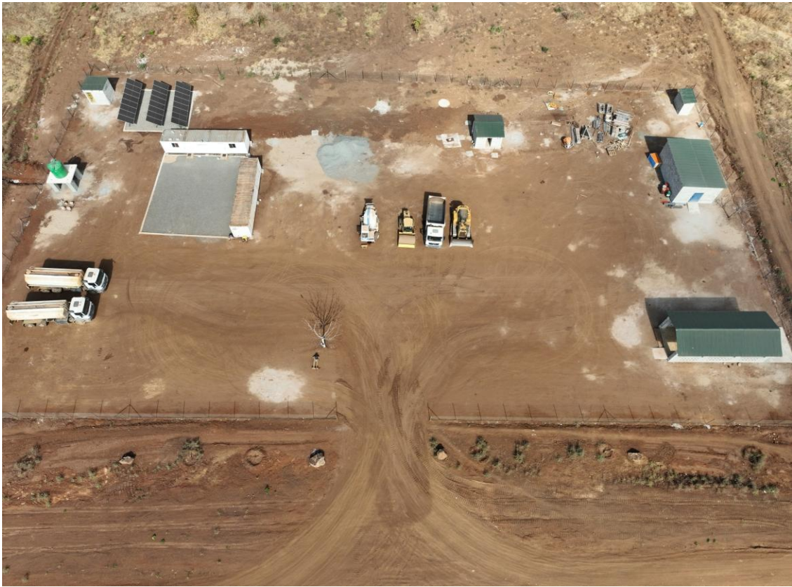
Picture 3. Contractors' laydown area at Kangankunde.
