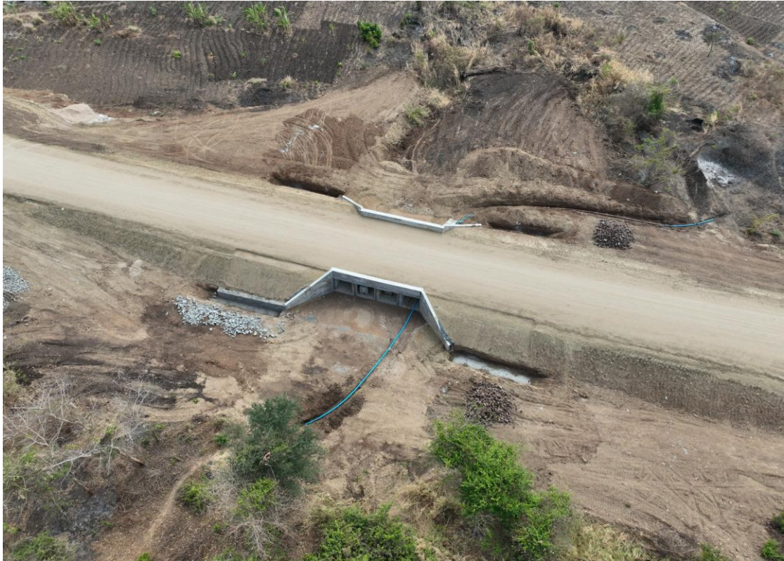
Picture 1. Completed culvert on site at Kangankunde.
