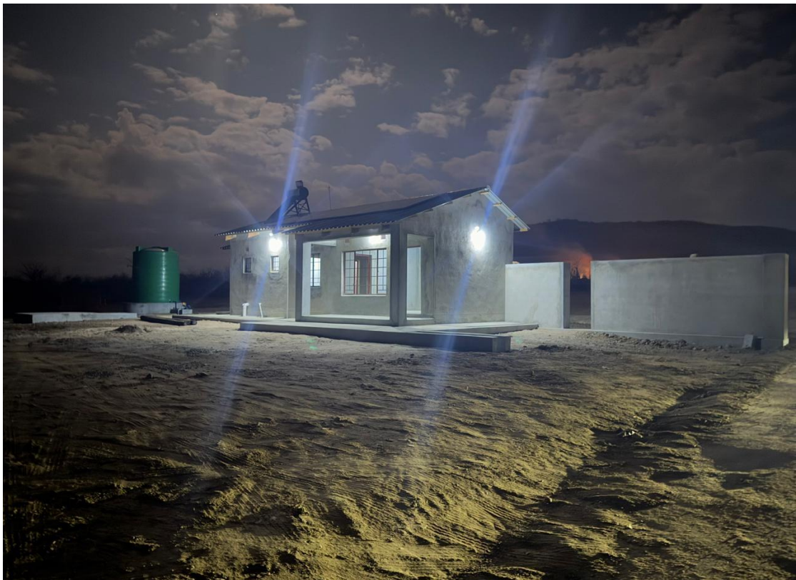
Picture 2. Security building at Kangankunde.
