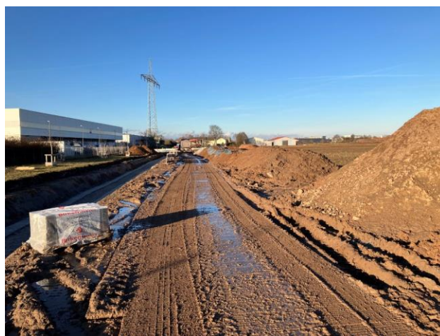
Figure 4: Preparatory works to install HV cable
