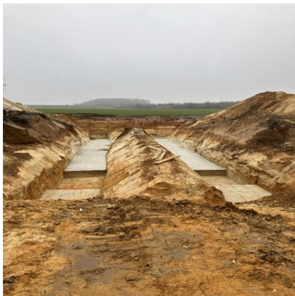
Figure 5 & 6: Concrete slabs as foundations for the duct pipes and start of installing the duct pipes (1.4m diameter) ICPP in December 2025
