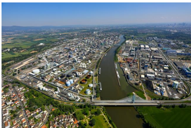
Figure 9: Infracore Park Höchst, Frankfurt
