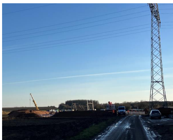
Figure 7: Earthworks at LEP site in December 2025
