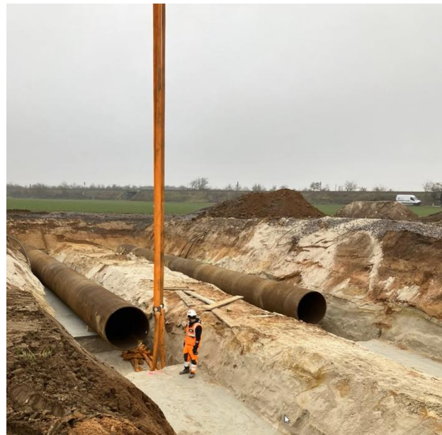
Figure 5 & 6: Concrete slabs as foundations for the duct pipes and start of installing the duct pipes (1.4m diameter) ICPP in December 2025
