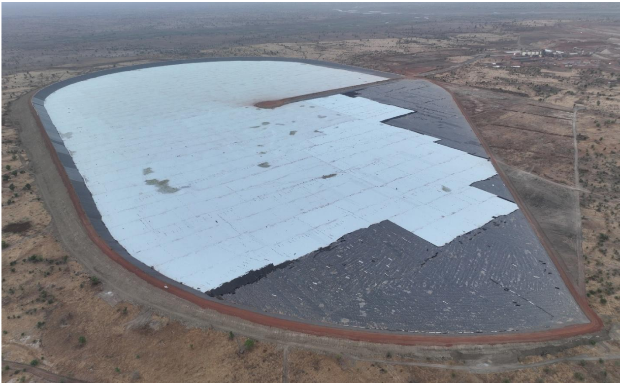
Photo 5: Kiaka tailings storage facility
