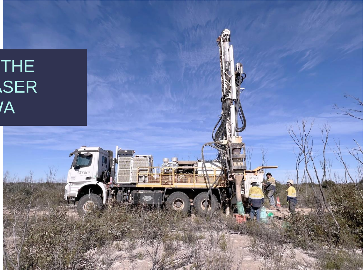
Exploring subsurface, air core drilling, May 2024
