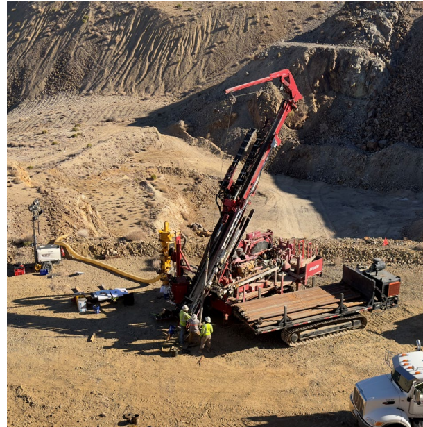
Extensions of pipes at depth
