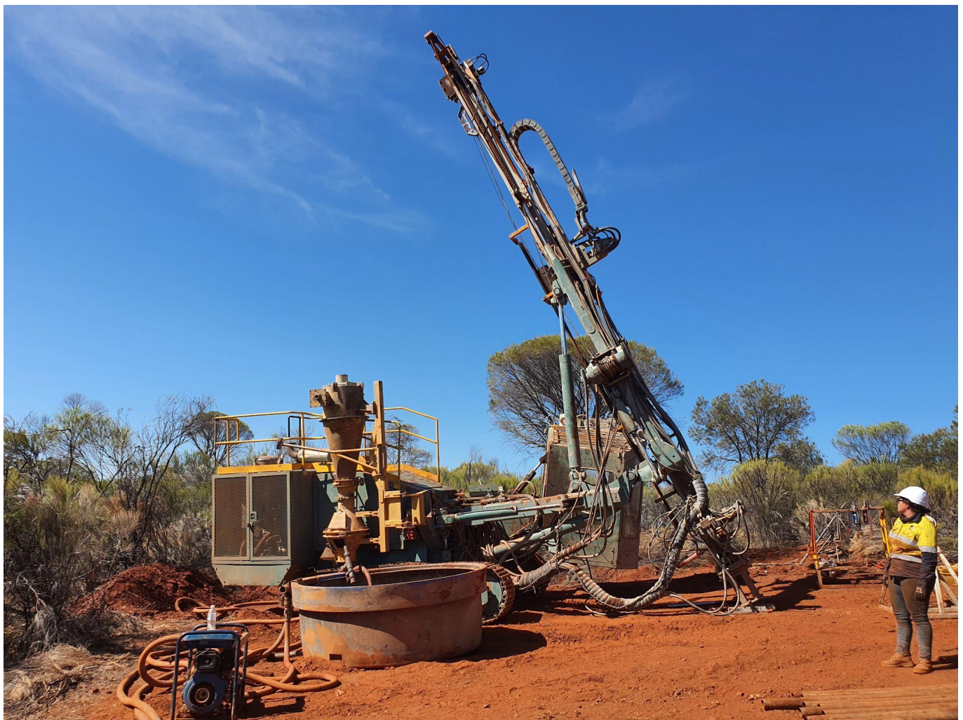
Figure 08: Drilling at the Euro Project
