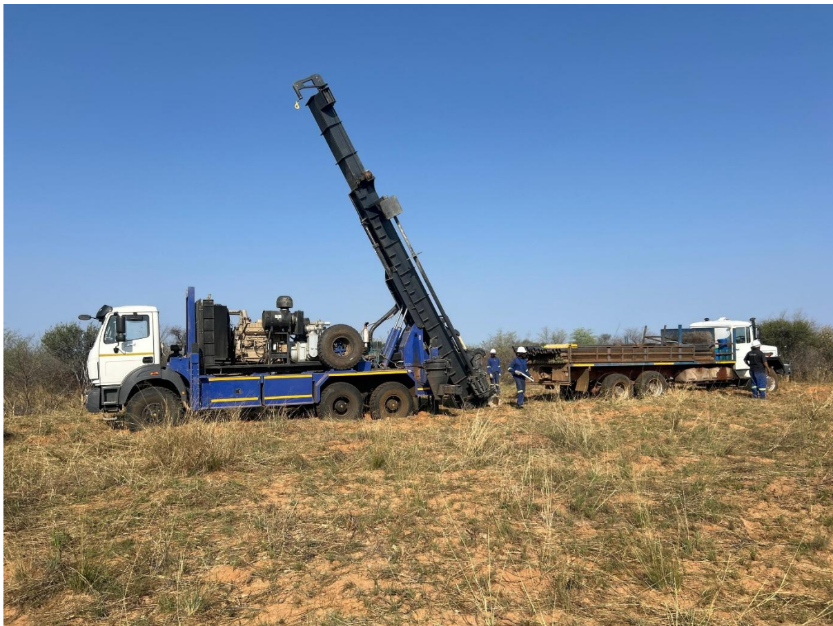
Figure 1: RC drilling commences at the Powerline Project
