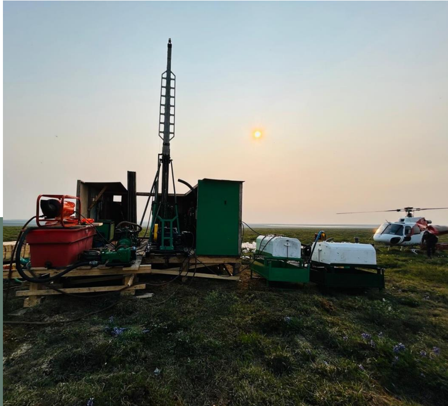
Diamond Drilling at Rae Project
