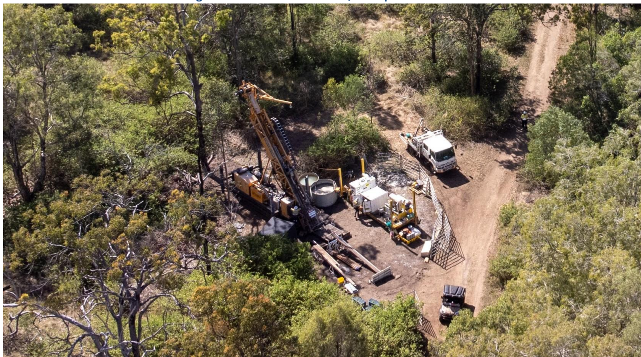
Figure 1 Drillhole 25BRD0037, 10 September 2025
