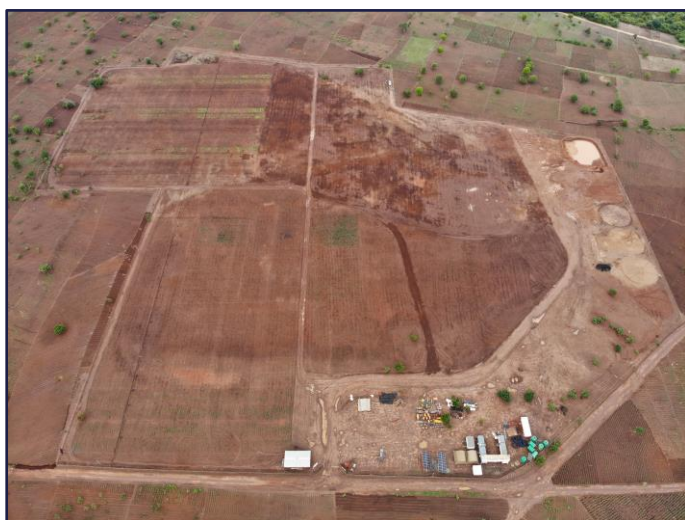
Figure 5: Rehabilitation site backfilled (December 2024)
